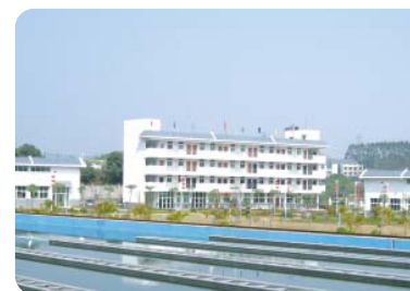
Water Plant(Drinking water)
