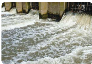
Sewage Treatment Plant
